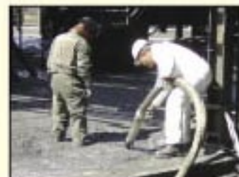
Operator adjusts pickup nozzle air inlet valve to supply the right amount of ambient air at nozzle inlet to entrain heavy sludge and drier material.
