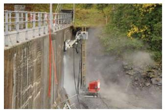
The operation width of the new power head can easily be increased and the traverse is easily extended for up to 4 m operation width. This feature is particularly advantageous for increased production on bridges and similar large surface projects.
