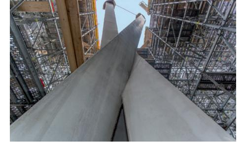
formwork solution that PERI developed consisted of a total of 82 3D-designed architectural concrete timber formers. They were mounted onto components of the PERI UP scaffold construction kit and finally sealed. The PERI UP Weather Protection Roof ensured that work could
