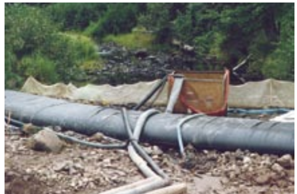
A rented submersible Flygt Bibo pump is seen here dewatering the pipeline trench.
