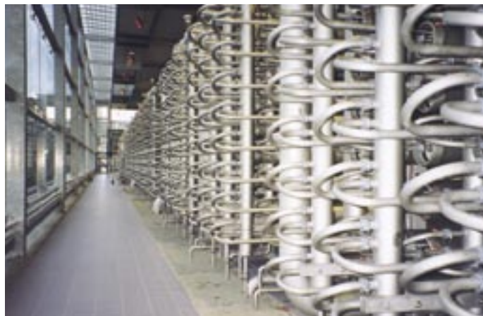
The Méry-sur-Oise world's largest nanofiltration plant for treating river water.
