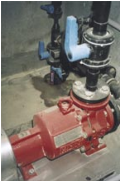
Plastic-lined magnetic drive pumps from ITT Richter, Kempen, dose the chemicals necessary for the CIP cleaning of the membranes.
