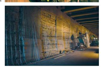
Operating at 1000 bar the Aquajet system is using a water flow rate of 260 l/min and is achieving a removal rate in the deteriorated concrete of up to 1,5 m<sup>3</sup>/h.
