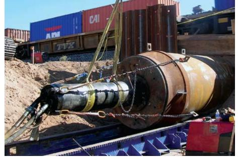
culvert when ramming in the new steel pipe, they did not have to change the drainage flow patterns. Also, there was never any fear of loss of integrity to the rail bed and embankment. They never had to worry about creating any voids during the installation since they were driving a solid steel pipe. Nor did they have to be concerned about any post-project settlement with pipe ramming.
