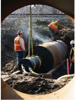
other in putting in new drainage pipe. With pipe ramming, there is no interruption of service, no appearance of settlement, and no concern about rail bed or roadbed integrity.
