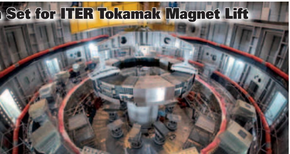
problem: how to lift the PF6 ring to its final position and bolt it to the tokamak structure within tight space constraints and without access to a crane," said Nello Dolgetta, in charge of the operation. "To raise the PF6 ring by 2 m, we are performing a synchronized lift to provide a safe and secure lift operation. Early trials with a dummy load were very successful."
