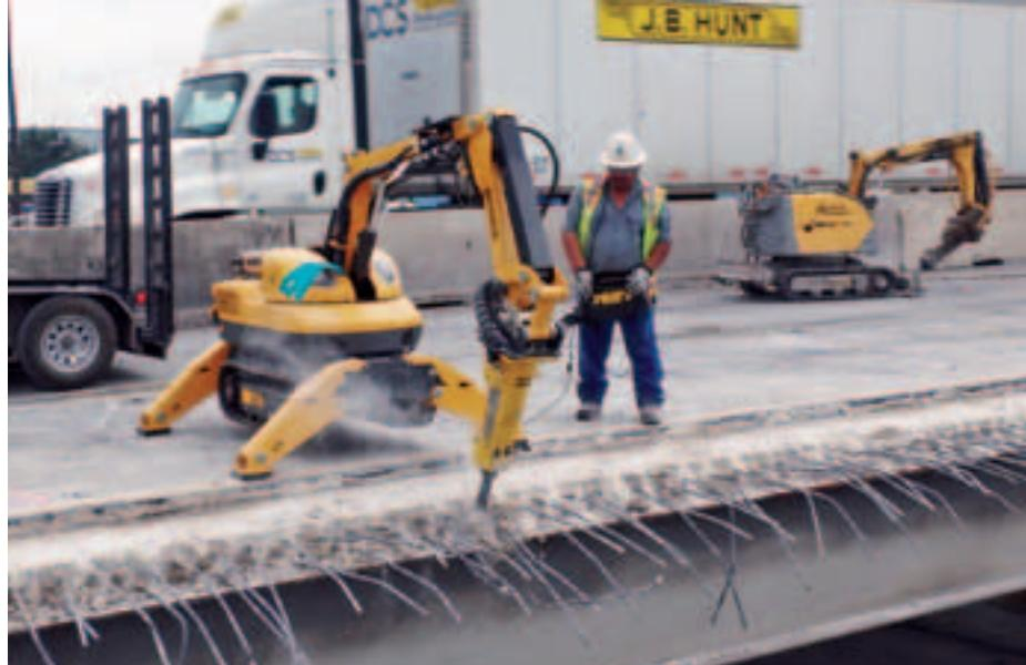
Remote-controlled machines drop labor costs by 33%, accomplish the job faster and greatly reduce the risk of injury. Plus, it is a lot easier to recruit young workers to run remote-controlled machines and hydrodemolition robots as opposed to handheld tools.
