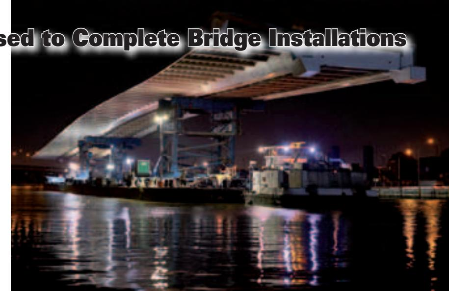
CS5000 has a 4,500 t capacity per tower and is still being used on projects today. For its smaller jobs, the team deploys smaller systems which can be handled manually and can be easily transported by road.
