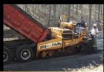
LorBoy 8516 25,000 be class 8' to 16' paver Curmins 130HP engine, Legen("\* screet system with 10% slope or extensions, variable speed 14" cast segmented augers, patented under auger cut-offs.
