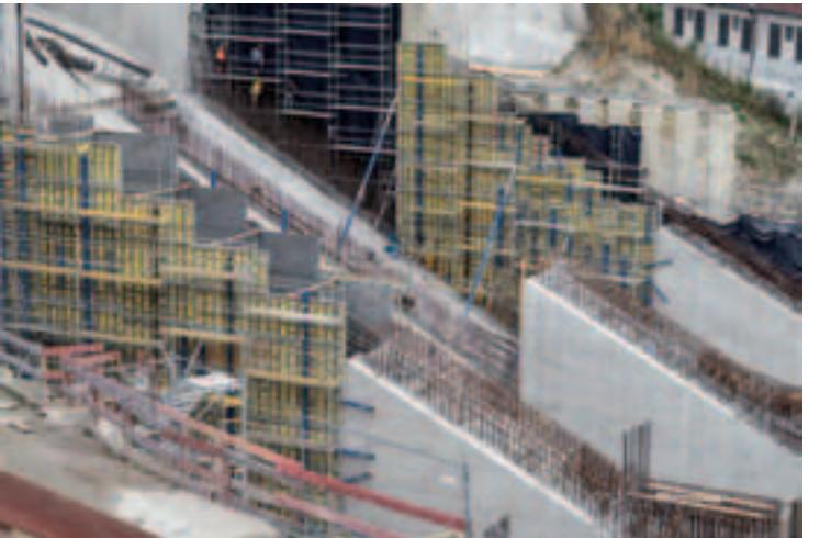
3D formwork planning is one of Doka's key disciplines, demonstrating that also slopes of almost 30° and slab thicknesses
