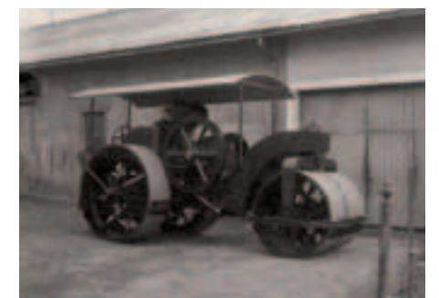
In 1911, HAMM launched the world's first motorized road roller. The Hamm brothers had already been making motorized machinery. They built stationary traction engines, motorized plows and threshing machines.
