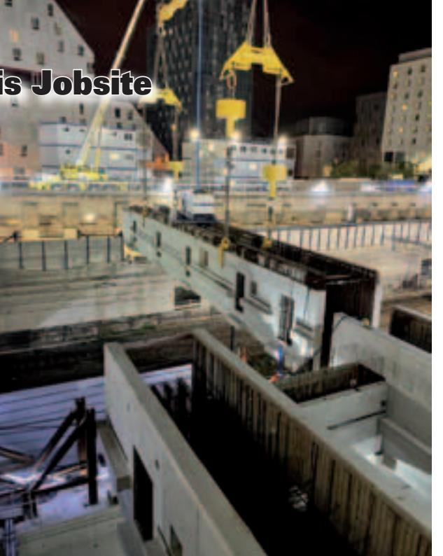
the SyncHoist's wireless operation allows us to evaluate and control the beam's stability, as well as achieving the precise
