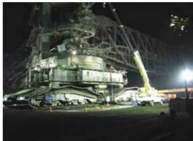
Enerpac synchronous lifting technology was chosen for lifting this 5000 tons coal mine dredger to inspect and refurbish the giant machine's slewing ball race, while monitoring the 2200 ton load's centre of gravity.
