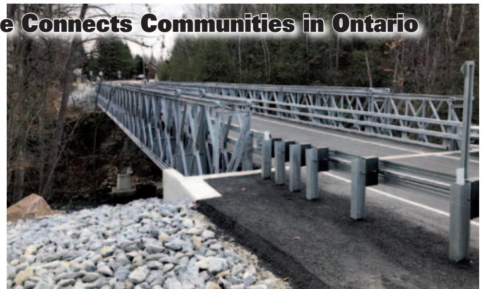
modular components, rather than large steel or concrete beam sections on narrow rural roads. Furthermore, it was estimated there would be reduced overall costs when compared to building with conventional reinforced concrete slab on steel or concrete girder systems.
