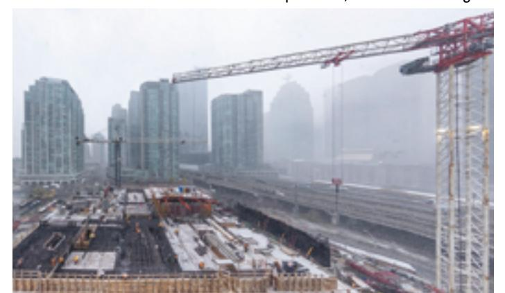
of material at the base of the construction site, led to the selection and development of the RCS Gallow (RCS G) Shear Wall System. PERI engineers offered a solution to hang all shear walls on the project off RCS G frames, enabling the formwork to remain in place at the top of the building at all times. This approach eliminates exposure of the formwork to the wind and time spent lowering formwork to the ground.
