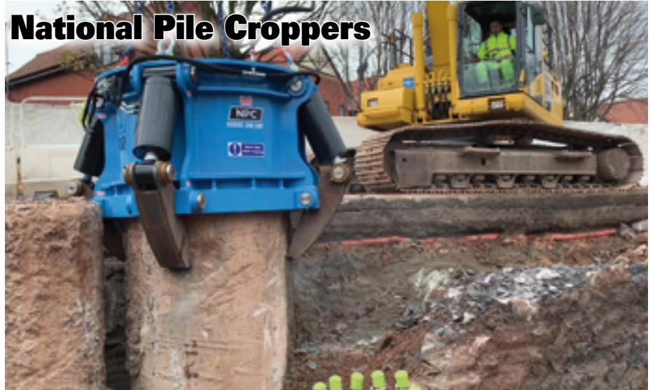
staff are at hand from the initial order to the installation on site to make sure that customers get what they pay for. Operation is still simple, with the cropper being lowered to the ideal height, with the jaws then being closed until pile sections 'pop' free. The broken pile section then can be easily removed for recycling to a dumper or a specified area," added Mr. Lee. "The feedback we've received has been beyond our expectations. Our customers seem to
