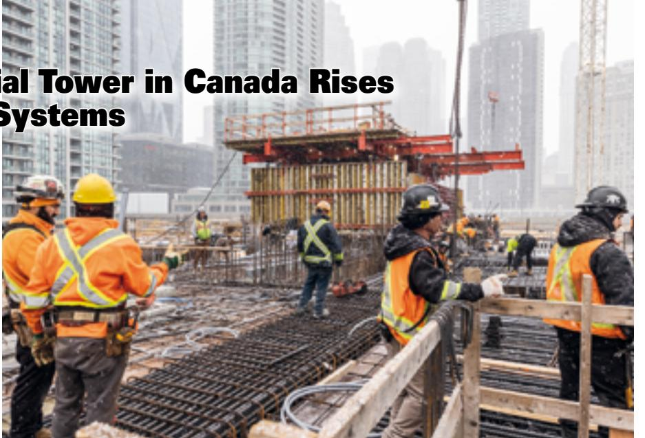
stair core to be raised from floor to floor without the use of the tower crane and with the minimum amount of labor. Due to the high capacity and flexibility of the system, only 6 hydraulic cylinders are needed for the task. This reduces the amount of cast in anchors into the structure to
