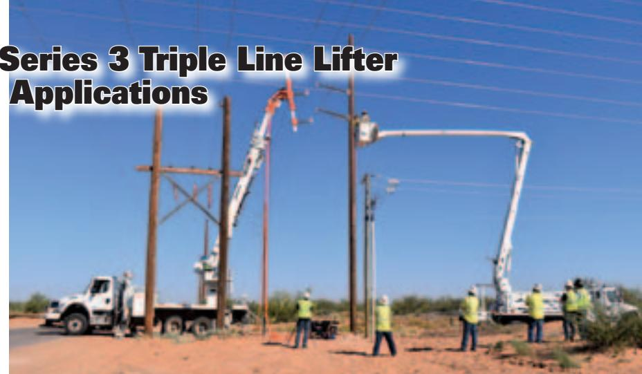
outside phases can also be extended to a maximum overall span of 4.8 m or retracted to a minimum overall span of 2.4 m. This feature allows the 3 phases to be positioned anywhere from 1.2 m to 2.4 m apart. Wear pads are installed within the assembly to maximize service life. A radio remote allows operators to control all hydraulic functions while working in a bucket.
